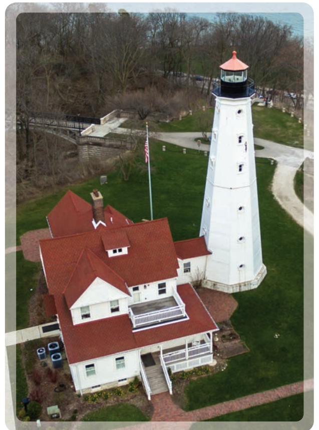
North Point Lighthouse
