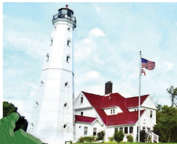
North Point Lighthouse
